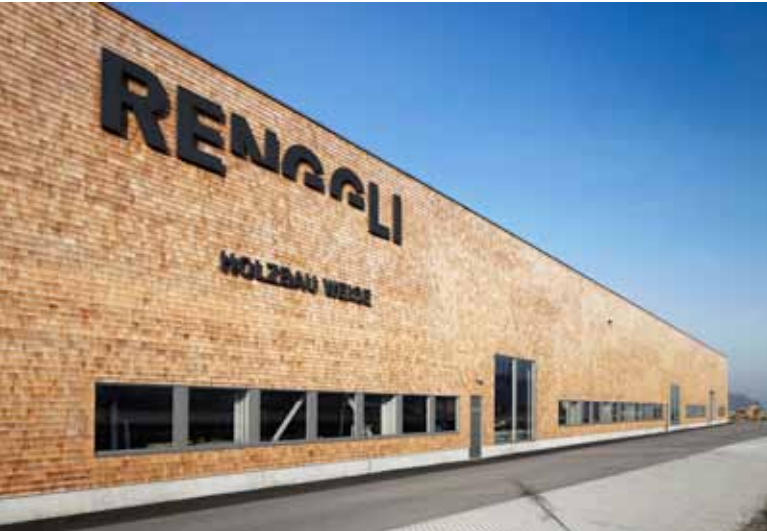
120 m long and certified by Minergie
